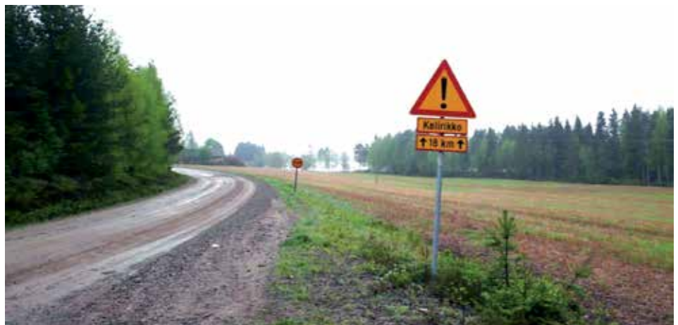
Figure 4: Truck weight restrictions are imposed every spring for low volume roads to protect road structure from excess damages due to wet pavement structure (Kelho, 2008).
