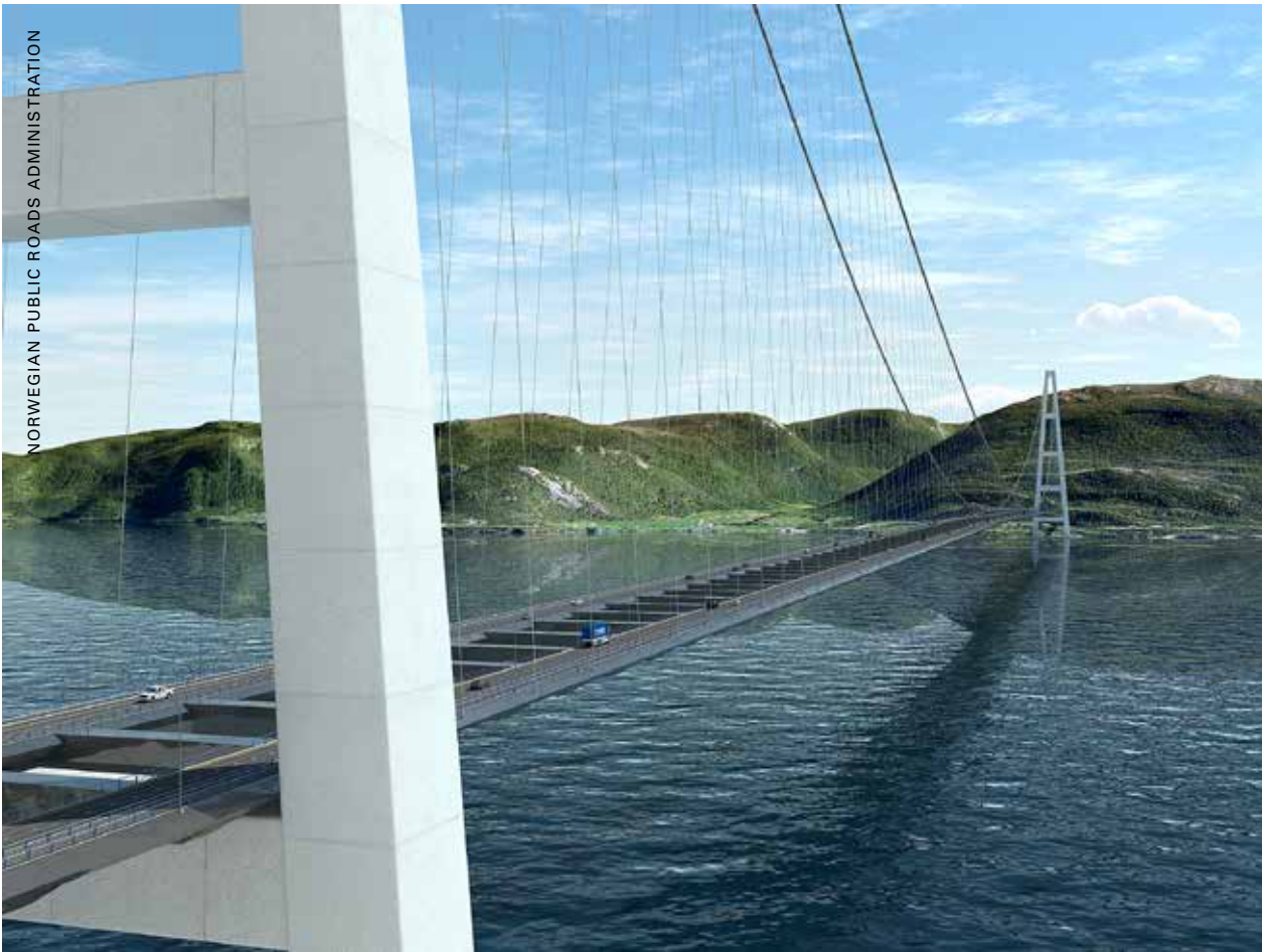
Suspension bridge with a midspan of 3,7 kms.
