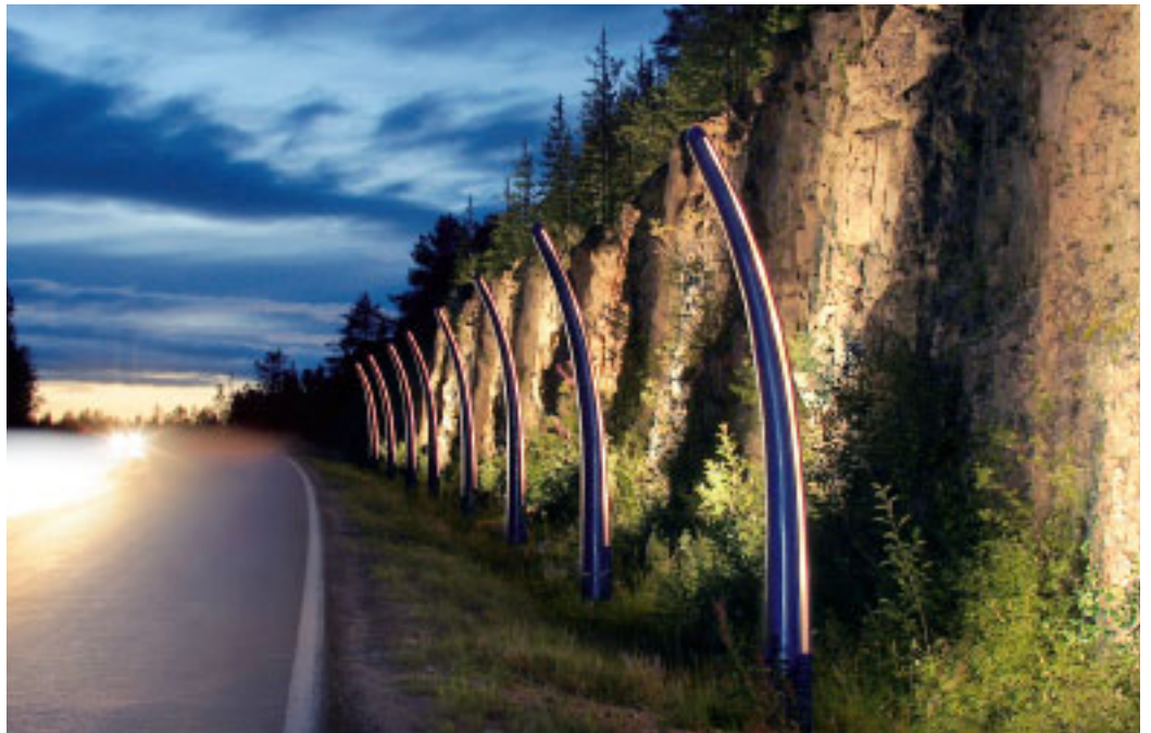
The light work in Muonio rock cut. Photo Jaakko Alatalo.
